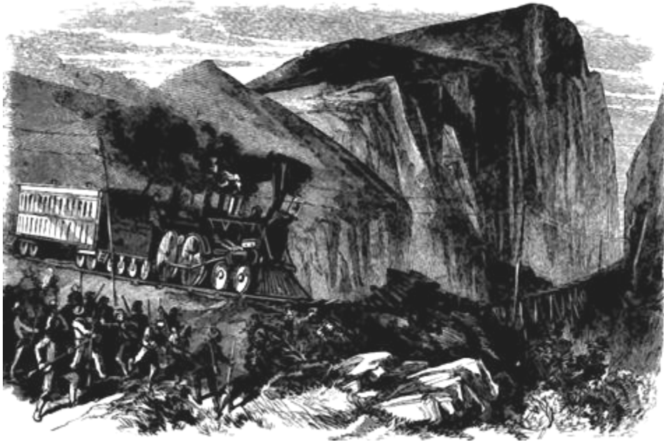
OBSTRUCTING THE TRAIN
